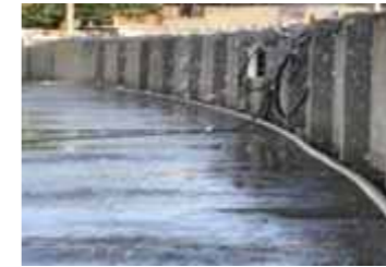
施工围墙自动喷淋
